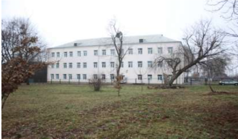
Building containing Dormitories, a Cafeteria and an Auditorium
